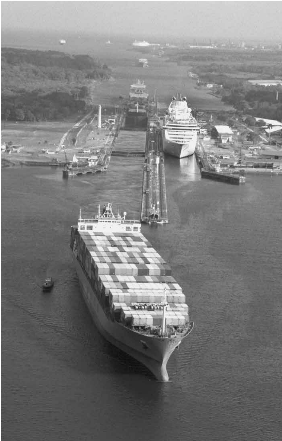
Figure 26.5 Gatun lock on the Panama Canal
