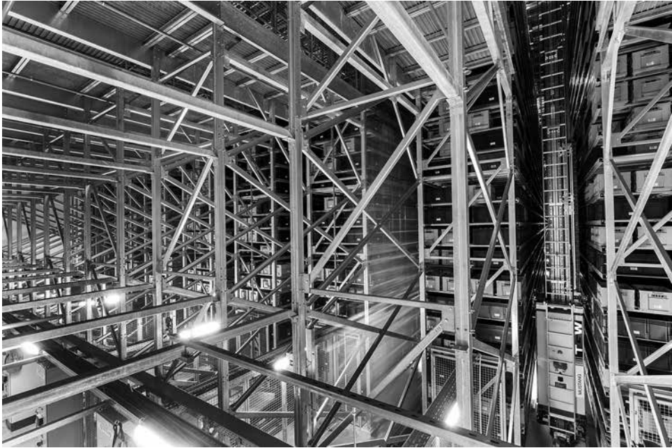
Figure 20.1 Miniload crane tote storage system
