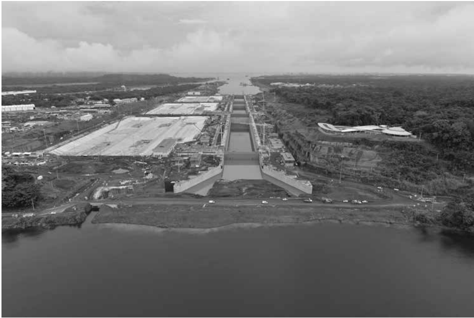
Figure 26.7 New Panama Canal locks under construction, 2015
